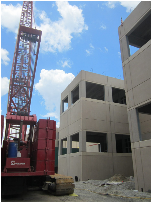
Above: Crane finished stacking the 500+ pre-cast cell modules on May 19.
