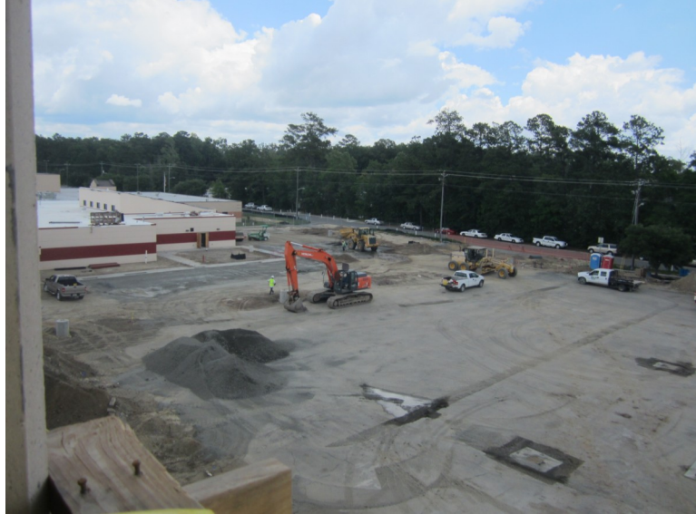
Left: The view from the top floor of one of the new inmate housing towers shows the parking lot being cleared and leveled for paving. The new employee parking lot should be completed in July.
